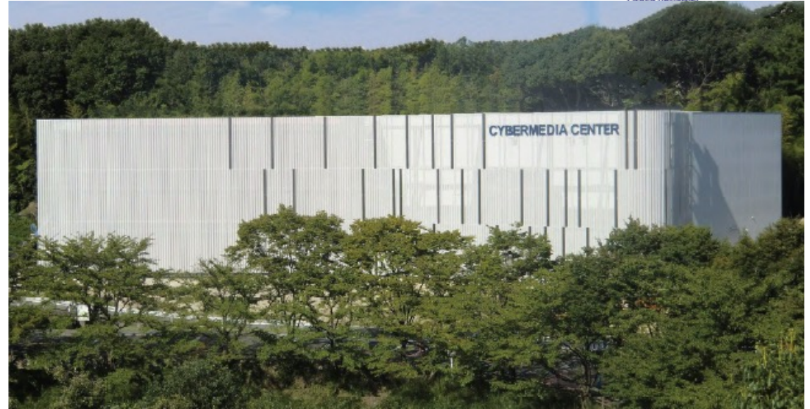
IT core as data center
