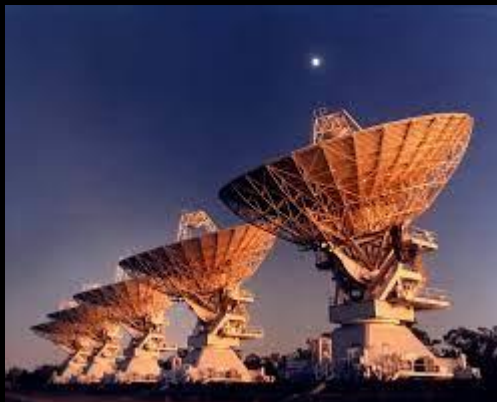
SKA Australia Telescope Facility
